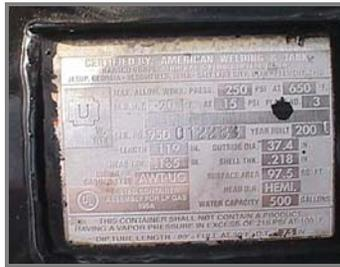
Figure 5.1.7d – Underground Tank Data Plate
