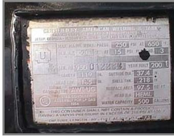
Figure 5.1.7d – Underground Tank Data Plate
