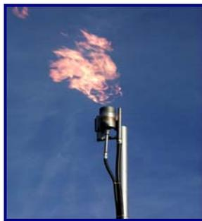
Figure 5.1.8d – Propane Burning from Flare Tower
